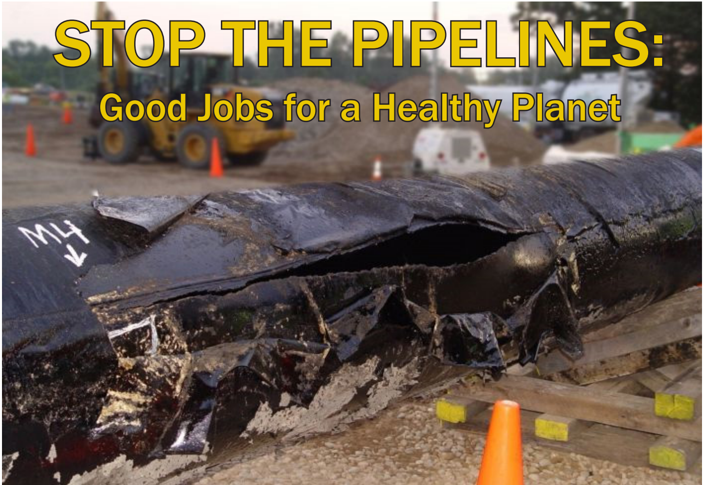
Ruptured Enbridge Pipeline
