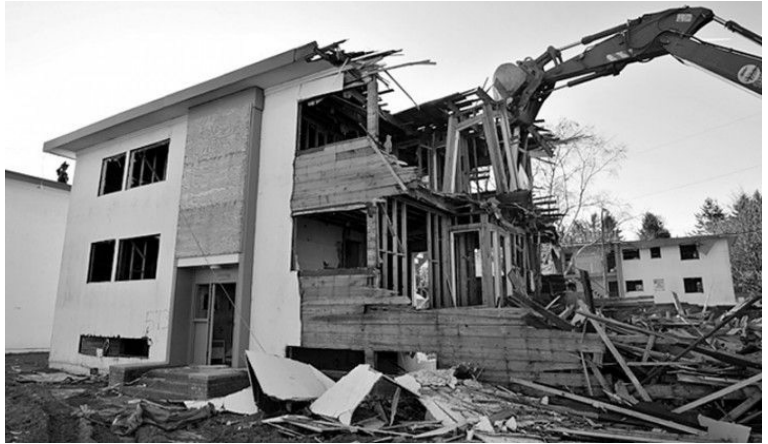
Demolishing Little Mountain Homes
