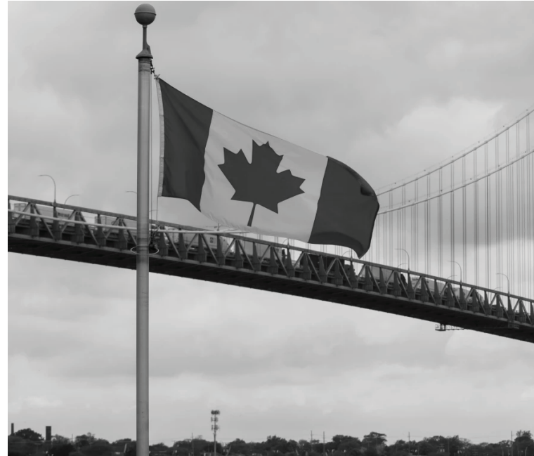
10,000 trucks cross the Ambassador Bridge between Windsor and Detroit e
