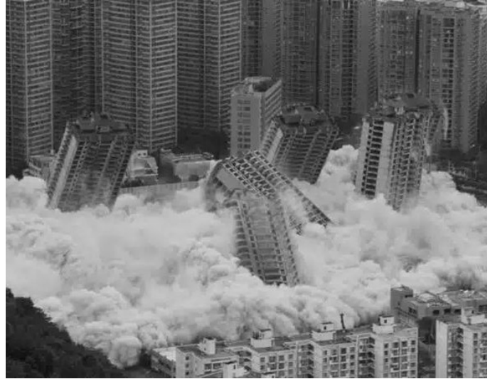
Unfinished apartments in Kunming were demolished
